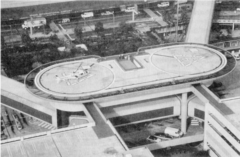
FIGURE 15-8 Heliport at Miami International Airport ( Howard Needles Tammen and Bergendoff & Miami International Airport ).
