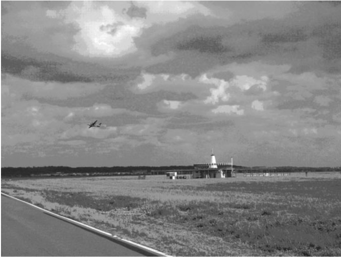
FIGURE 3-10 VOR beacon on the airfield at Ronald Reagan Washington National Airport.
